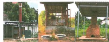
Figure 13: Examples of single chamber and brick incinerators
