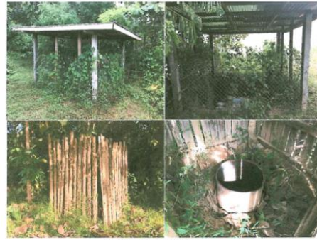
Figure 19: Examples of controlled bury pits in health facilities in Luang Prabang
